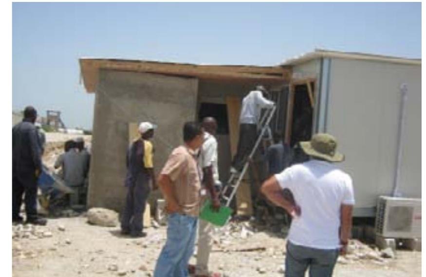
Navin Tuladhar overseeing the construction of the staff camp
