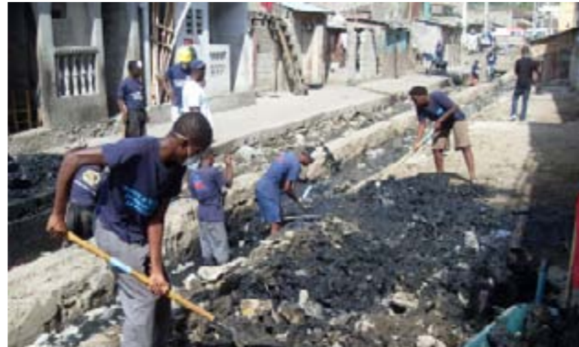
OJVC cleaning gutters in Shada 1
